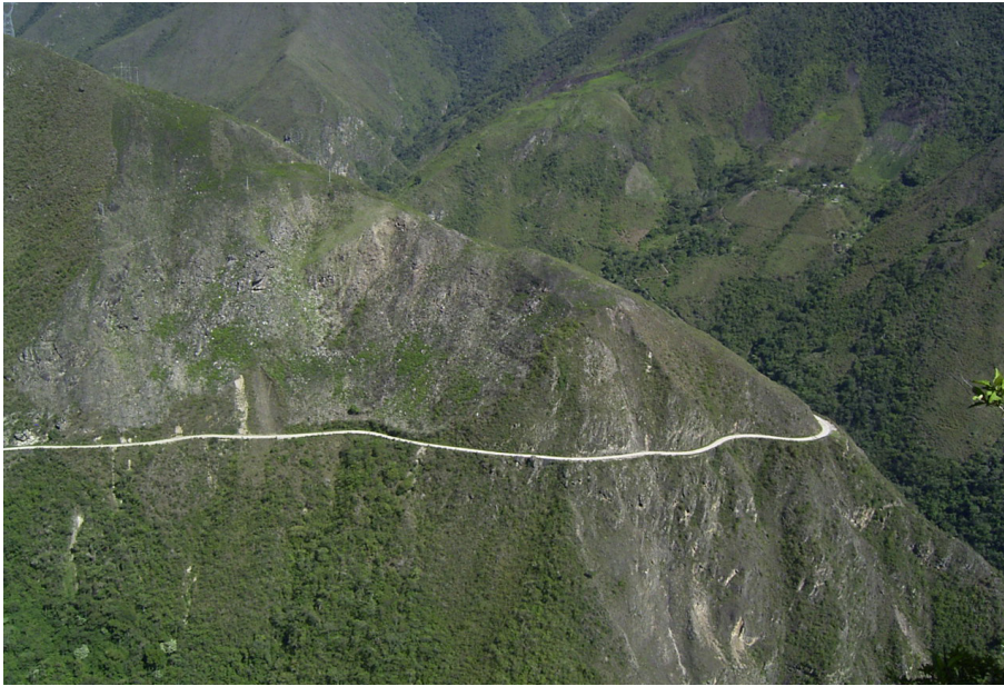
Traces of a fascinating past. There are still many signs of the rich and highly developed Inca culture in Peru. In such world heritage areas, modern activities require that a great deal of care be taken. This picture shows old Inca tracks on the side of the mountain by Statkraft's Cheves facility.
